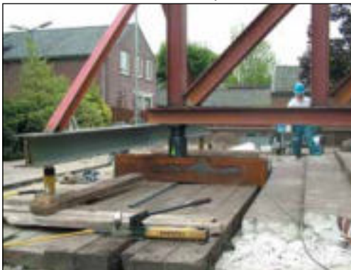
▼ P392 in action with RC256 cylinders.
