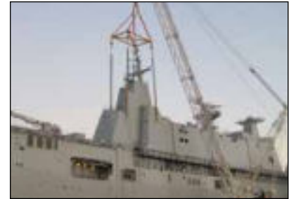
Synchronous hoisting and load positioning
