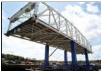
Incremental bridge lifting
