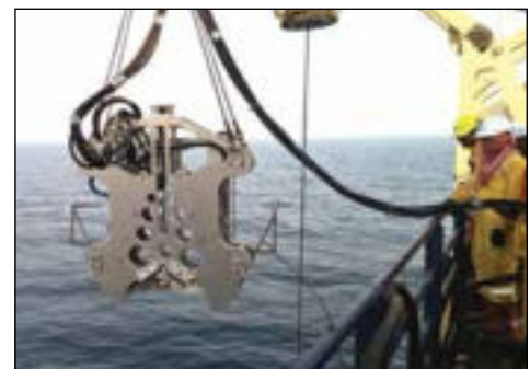
▲ MDWS Diamond Wire Saw lowered into sea.
