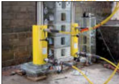
Bridge lifting and launching
