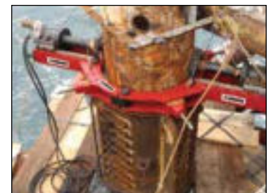
▼ DDU1636 casing pin drilling.
