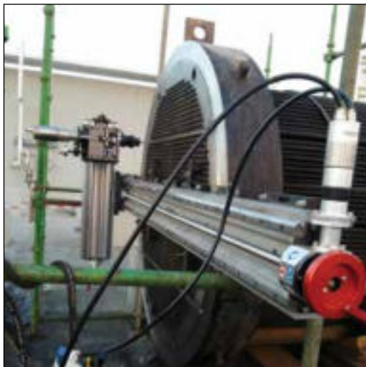
▼ MRY Milling machine on a heat exchanger.
