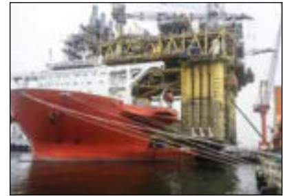
Synchronous superlift and launch
