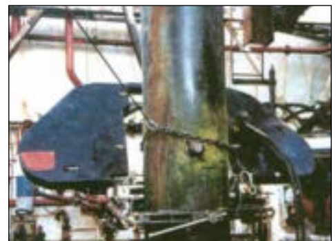
▼ Decommissioning job with band saw.
