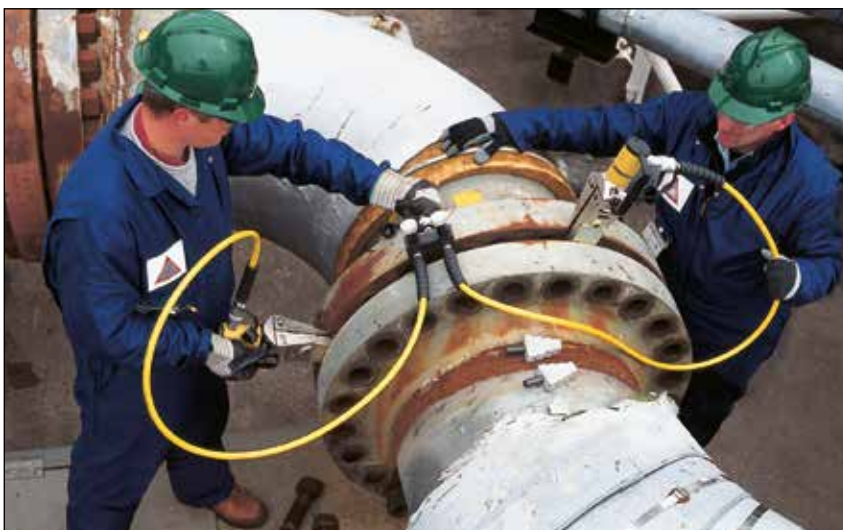
▼ Two FSH14 spreaders used simultaneously with Enerpac handpump, hoses and AM21 control manifold.
