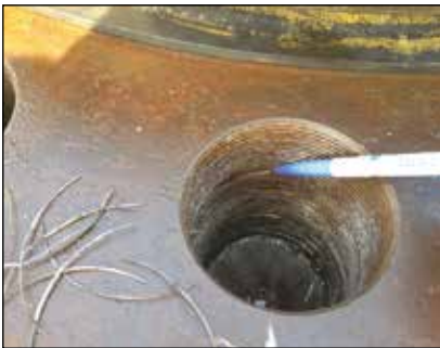
▲ A typical thread before refurbishment
