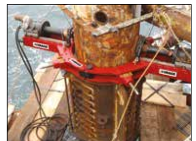
▼ DDU1636 casing pin drilling.
