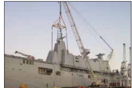
Synchronous hoisting and load positioning
