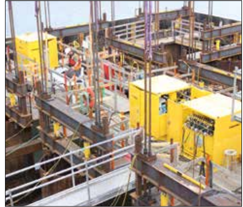
▲ Custom hydraulic pumps for a bridge deck launching system.
