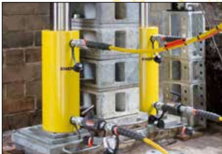
Bridge lifting and launching
