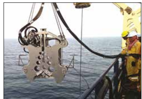
▲ MDWS Diamond Wire Saw lowered into sea.
