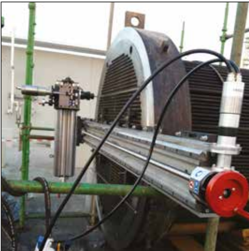
▼ MRY Milling machine on a heat exchanger.
