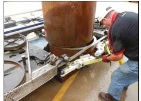
▲ Pipe cutting with BS portable band saw.
