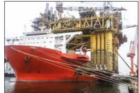
Synchronous superlift and launch
