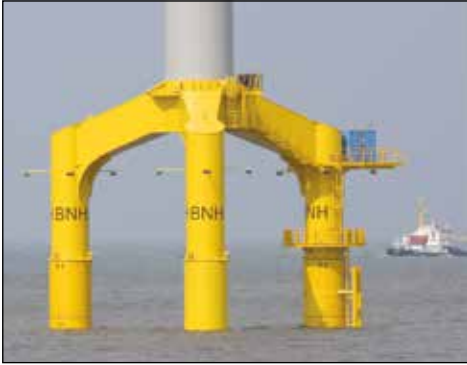
▲ Offshore wind turbines levelling: Enerpac's synchronous lifting system was the solution for levelling support cross pieces on 80 wind turbines.
