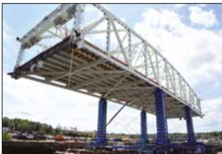
Incremental bridge lifting
