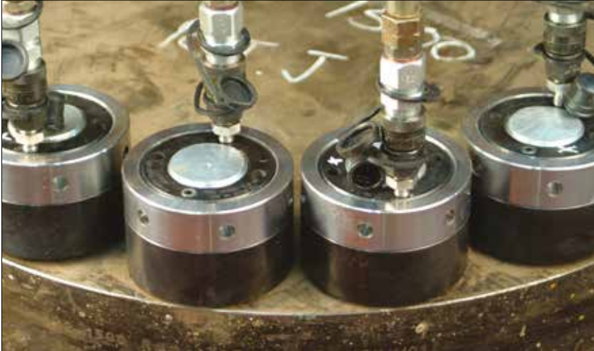
▲ Tensioning with hydraulic nuts.
