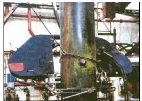
▼ Decommissioning job with band saw.
